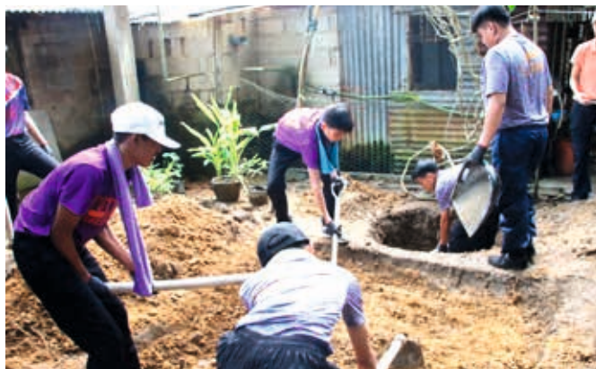
Students designed and built piping systems for the community
